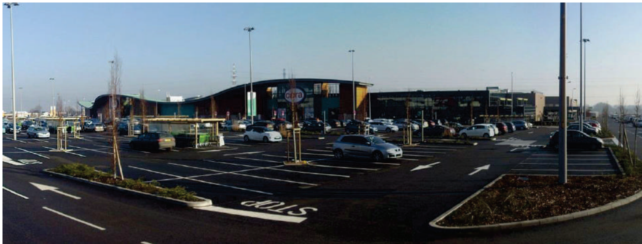
Figure 179 : Le centre commercial Cora
